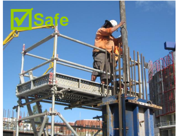
Figure 5 – Pouring concrete into column form. Good access provided.
