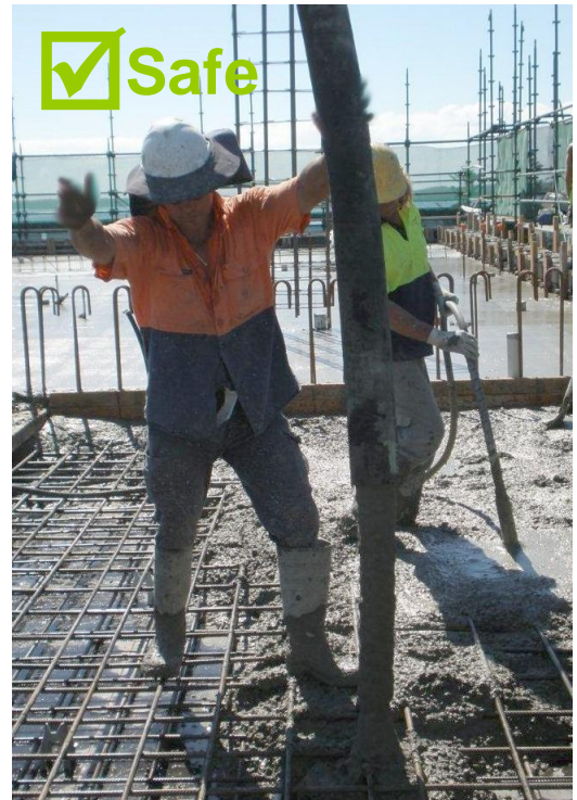
Figure 3 – Line hand guiding hose and signalling to pump operator.
